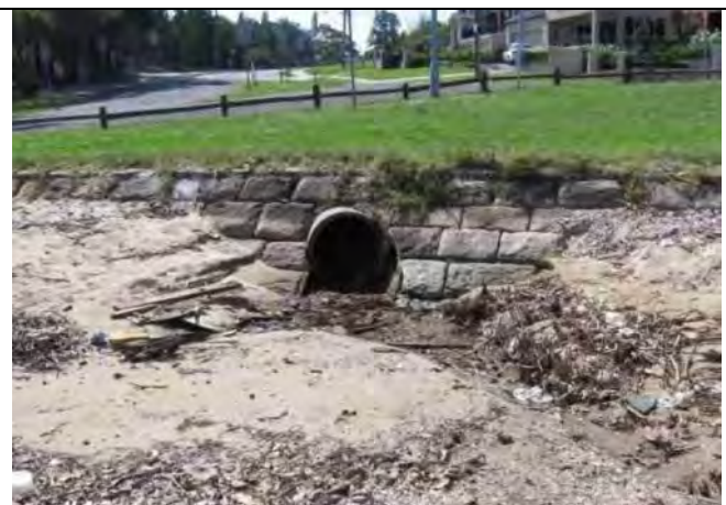
b) Sedimentation, scour and organic matter around outlet, Kissing Point Bay (source: AECOM, 2010).
