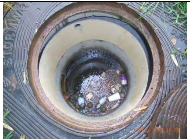
b) Continuous deflection separation device, Clarkes Point.
