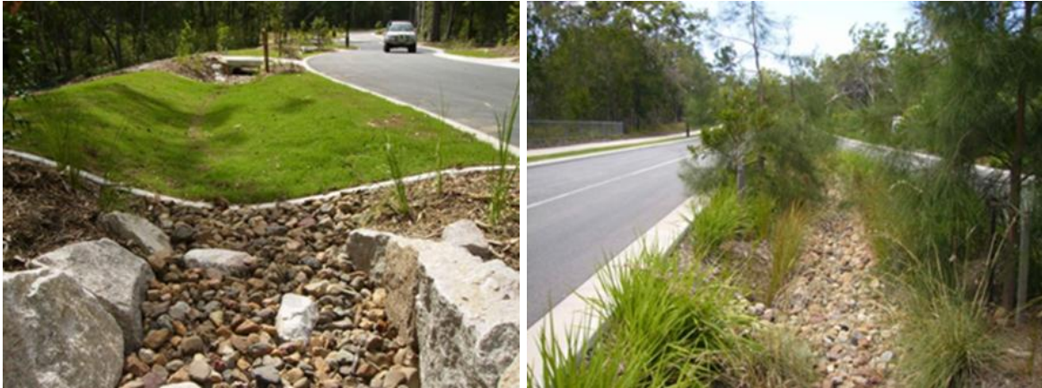
Figure 12-2: Examples of Grassed and Vegetated Swales
