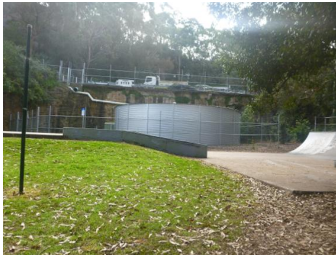
Figure 12-6: Existing Stormwater Tank at Blackman Park
