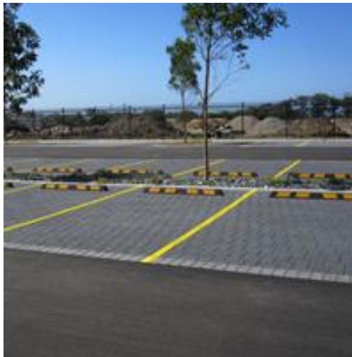
Figure 12-5: Porous Pavers at Sydney Water's new Potts Hill offices
