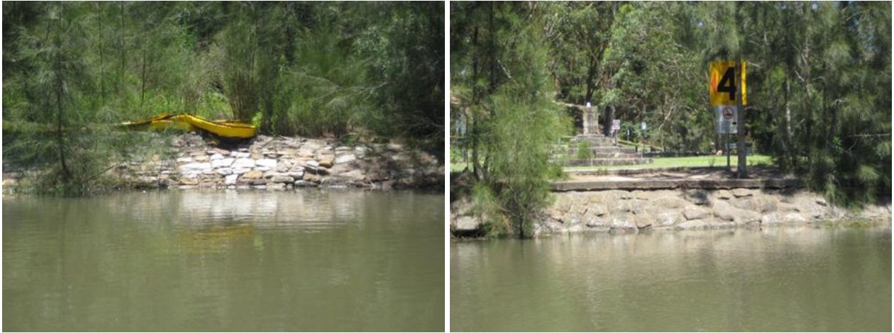
Figure 7-4: Seawalls along Middle and Upper Lane Cove River (Field visit photos)
