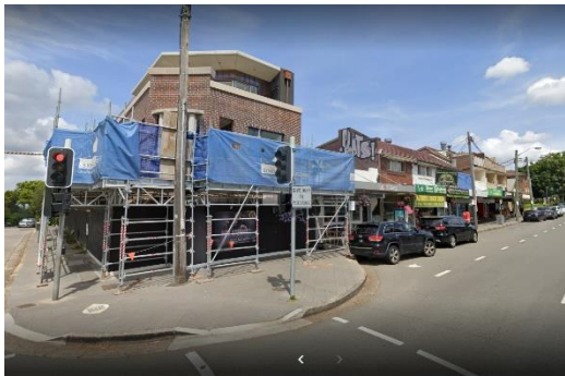
Figure 22 Boronia Park Shop-top housing development under construction
