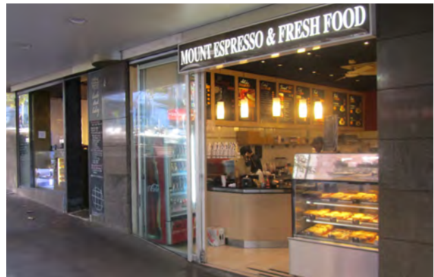
Photo A1.2. Visual and physical connectivity between the inside and outside creates active frontages.
