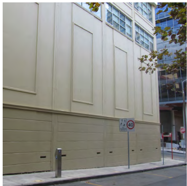
Photo A1.4. Blank walls are inactive frontages.
