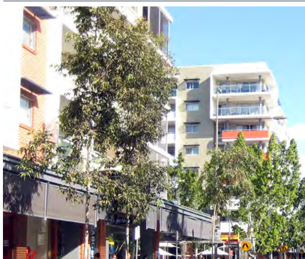
Photo 4.13. Separations between adjoining façades that incorporate windows and/or balconies should be consistent with Environmental Planning Policy No 65 and associated Guide.
