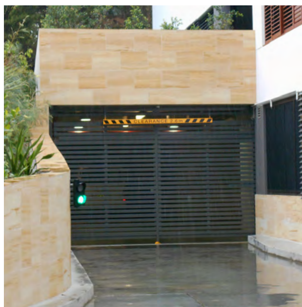
Photo 4.14. Visual impact of underground car parking entries is to be minimised by using roller doors or screens.
