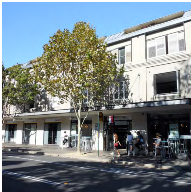
Photo 4.1. New buildings can maintain and enhance the scale and form of the predominant two to three storey linear street wall.
