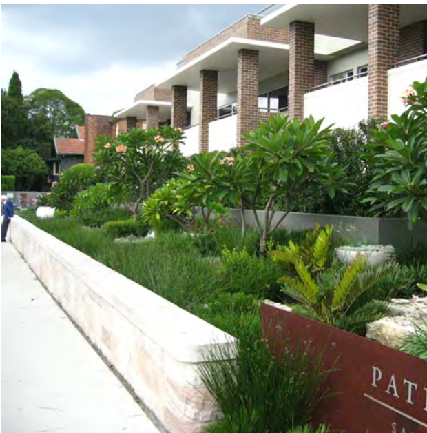
Photo 3.3. Development should contribute to enhanced pedestrian pathways and greater visual cohesion through the provision of consistent street setbacks suitable for deep soil planting of canopy trees.
