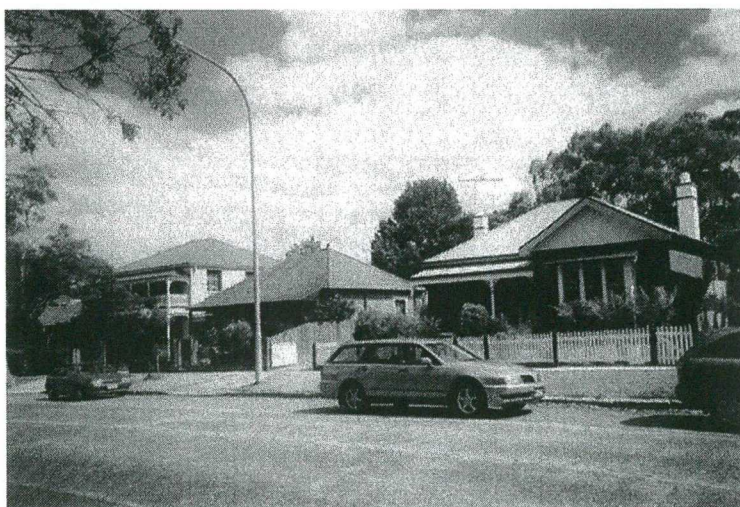
The group of freestanding cottages situated on the north side of Gladesville Street (no. 32, 34 and 36).
