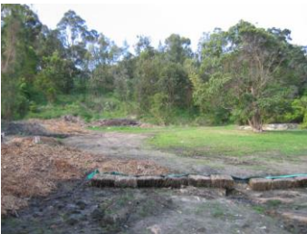
Stormwater outfall is impacting this area
