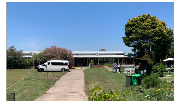
3 Non-compliant accessible parking
