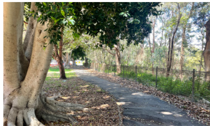
1 Existing path network requires remedial work
