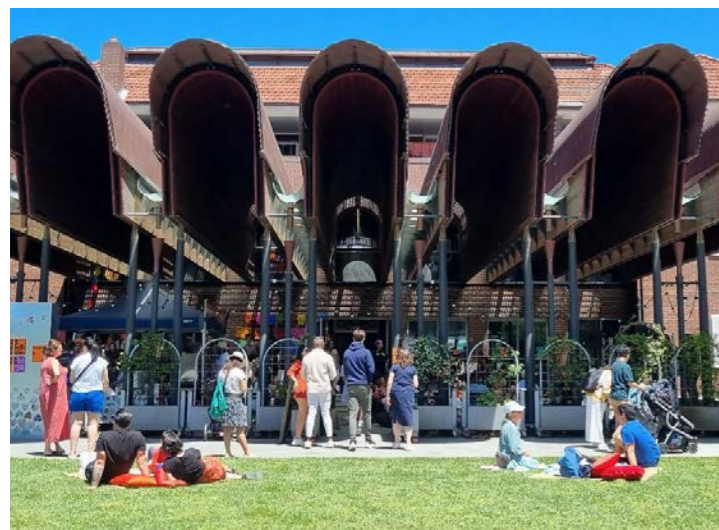
Joynton Avenue Creative Centre, Peter Stutchbury Architecture
